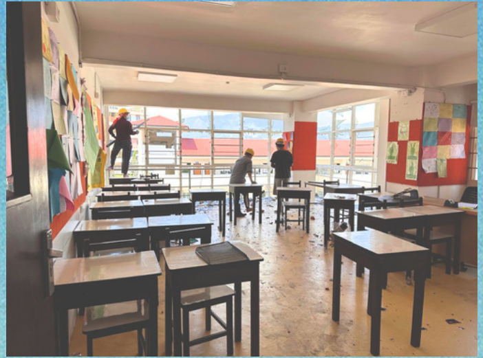
Cleanup and reconstruction underway
